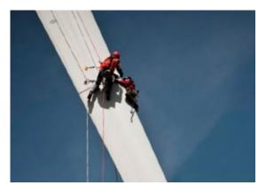
The rotors of the wind turbines must be regularly released of deposits that could negatively influence the aerodynamic behaviour of the complete system and with that the energy output. Our special cleaners not only clean effectively, they are also biodegradable, which is for example indispensable for offshore stations on high seas. OKS supplies a wide range of of biodegradable products, not only for the cleaning of wind turbines.
